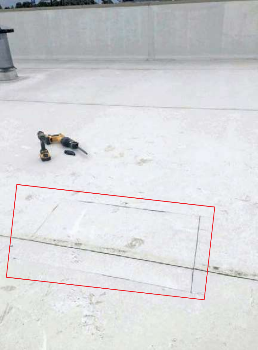
Figure 1 – Typical 2- x 3-ft. field sample.
