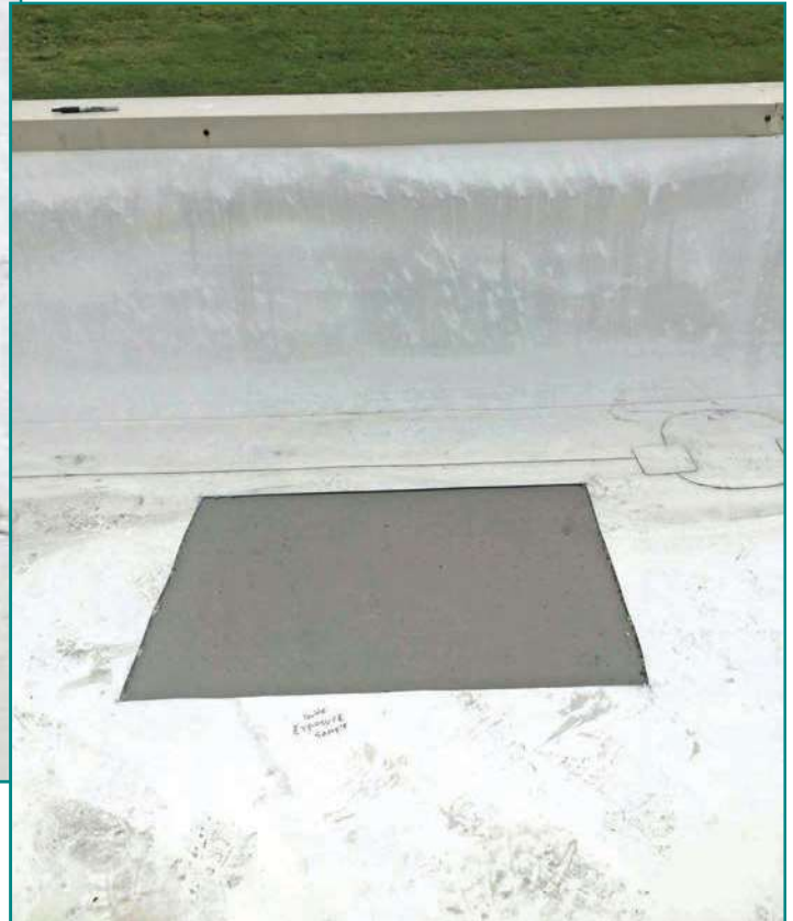
Figure 2 – Typical north parapet, 30 inches in height.
